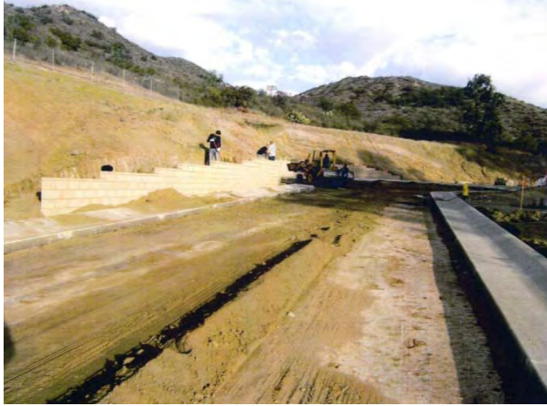
Figure 53. Allers Development Retaining Wall.
