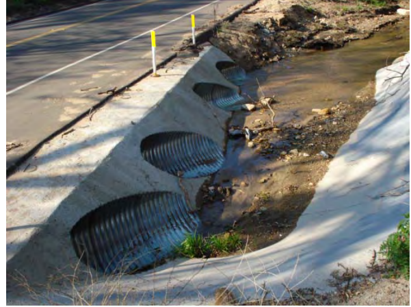
Figure 52. Culvert Built to Prevent Flooding.
